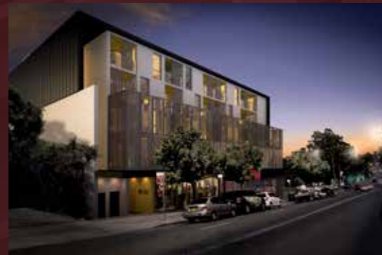
Alpha Apartments 46-50 Dunmore Street, Wentworthville 68 x 1 & 2 bedroom apartments
